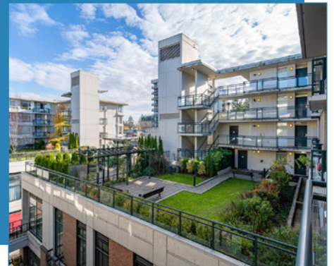
Rooftop common open space
