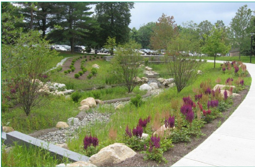
CENTRAL RETENTION POND ON LARGE PRIVATE DEVELOPMENT
