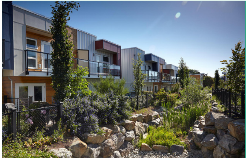
CENTRAL STORMWATER CHANNEL ON TOWNHOUSE SITE
