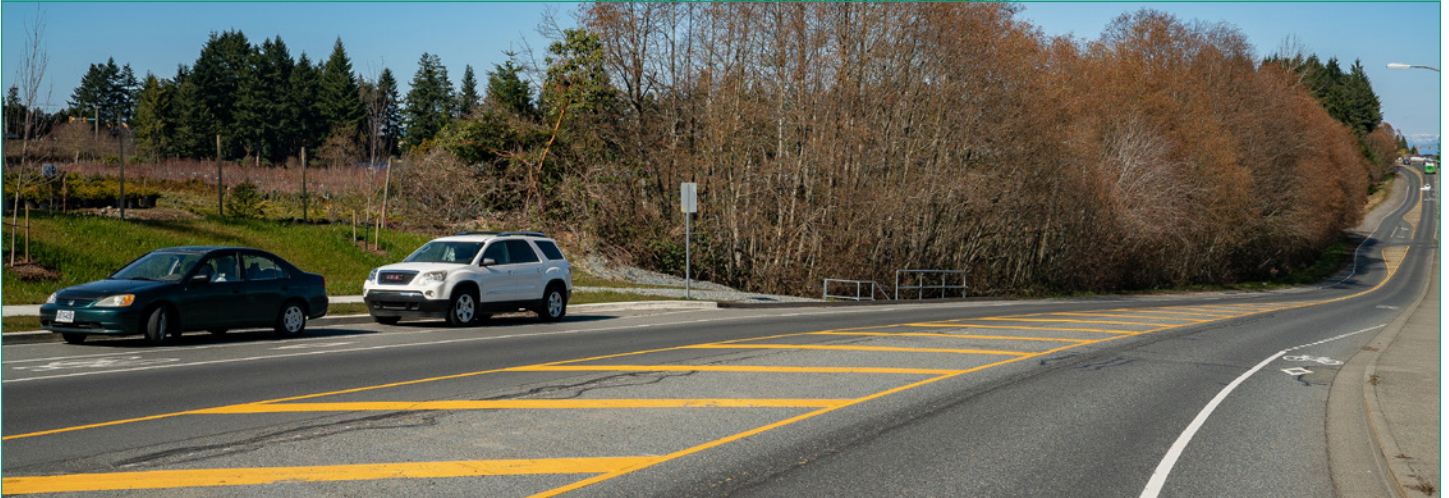
VIEW OF EASTERN BOUNDARY OF SITE ALONG UPLANDS DR., LOOKING NORTH
